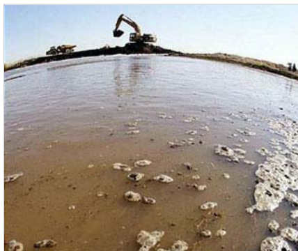
A BACKHOE breaches a levee Thursday at the Eden Landing Ecological Reserve in Hayward, allowing nearly 200 million gallons of Bay water to rush into a 300-acre dry former salt pond and restoring it to tidal marsh. (JANE TYSKA - Staff)
